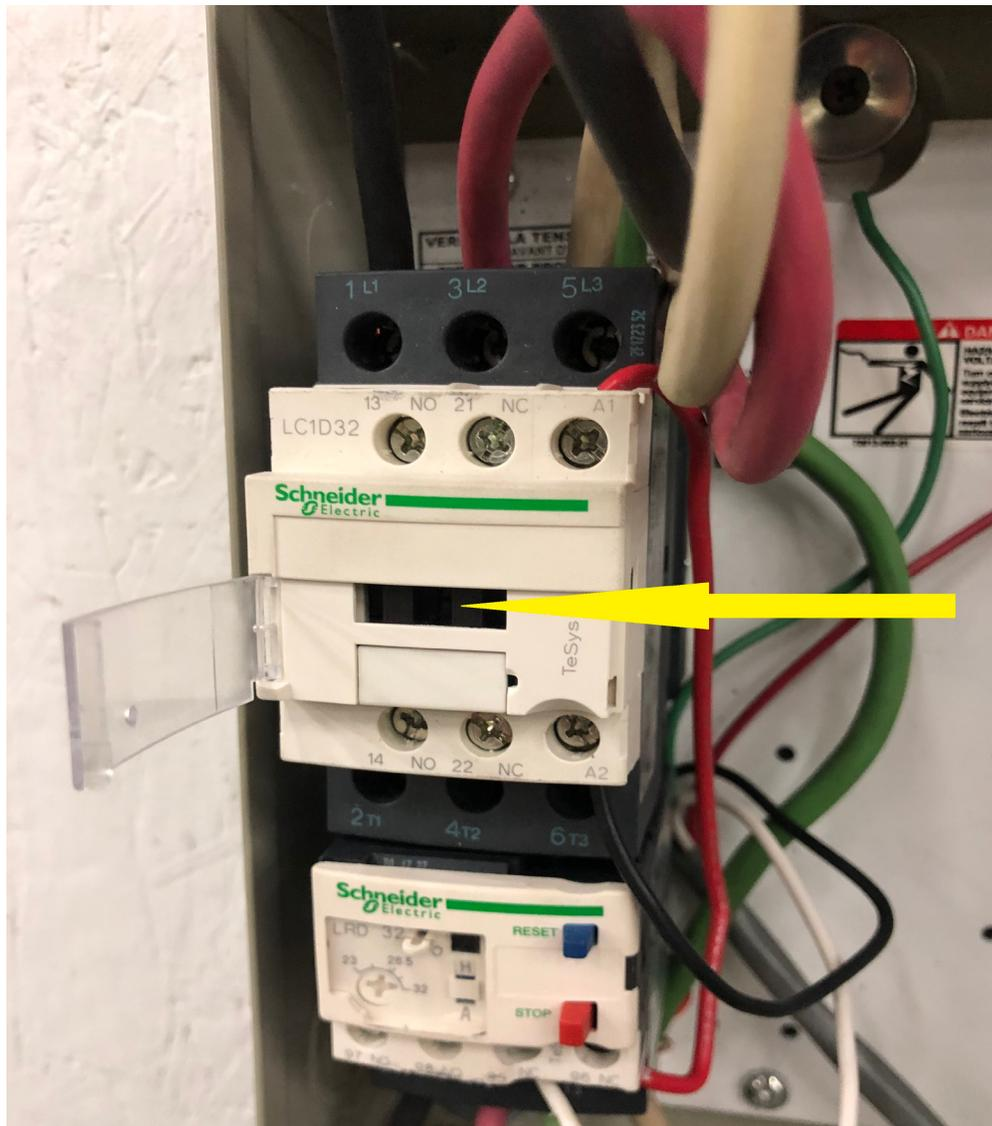
2) The customer can also use a voltmeter to test the voltage at the terminals at the top of the starter. Have the customer put the voltmeter in voltage mode for AC power. The usually looks like V~ (V with a wave). Between any two legs (i.e. L1 and L2) there should be between 208 and 240 volts.
