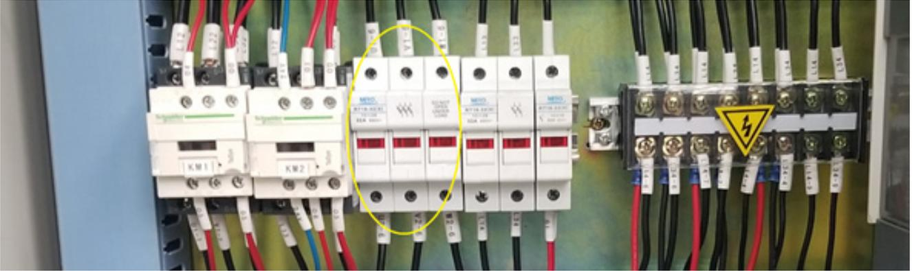
Otherwise, a voltmeter will be need to test for continuity on the fuse block.
